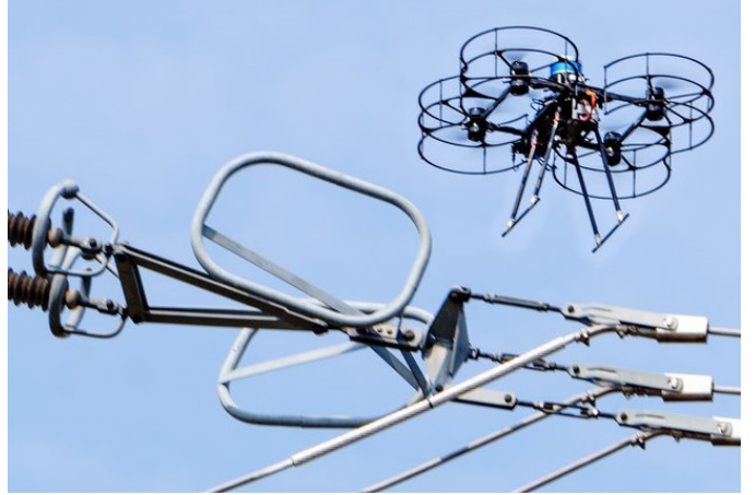
Figure 1. UAV performing visual inspection on a power transmission line.
